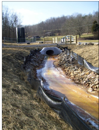
Treated water leaving the Thomas Fork Doser, before entering the creek.
