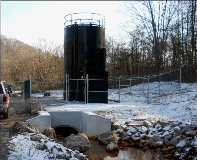
The Thomas Fork Doser Project is the first step in reclamation goals for the stream. Next Hysell Run will be addressed.
