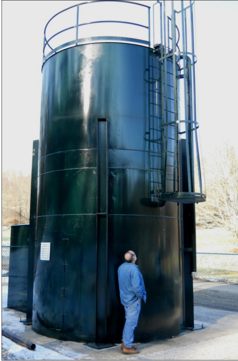
Steve Jenkins, Meigs SWCD Program Administrator, demonstrates the height of the doser silo, which will hold a maximum of 35 tons of lime material.
